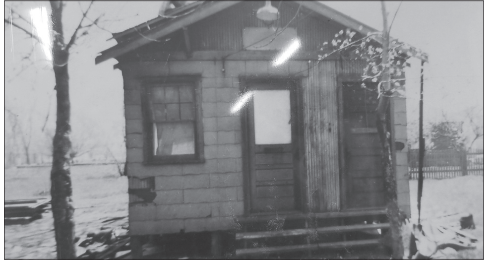
Forest View's first village hall near 4500 S. Maple Ave.
